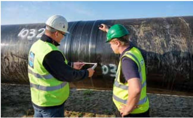
Figure 5. Quality inspection of the overlap width.
