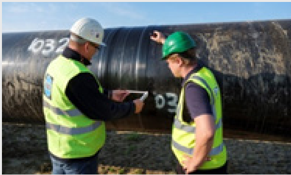
Figure 11: Quality inspection of the overlap width
