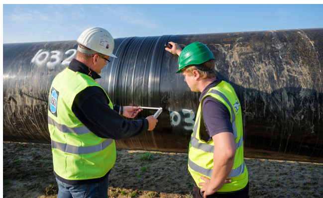
Figure 5. Quality inspection of the overlap width.
