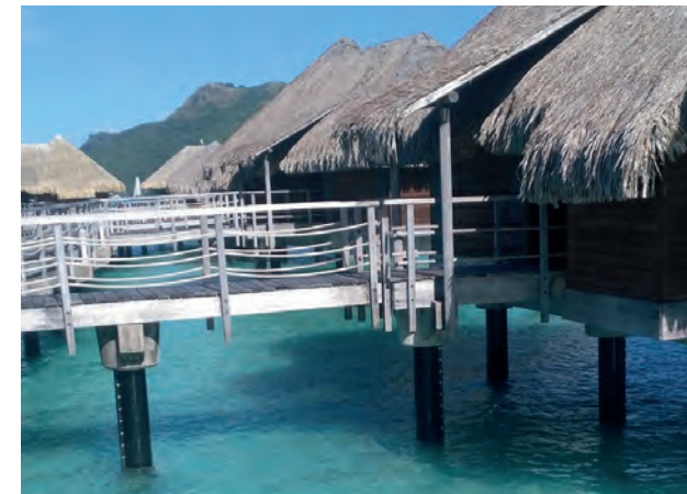
Polinesia Francesa MarineProtect®-2000 FD 1.019 pilotes, DN 300 (12")
