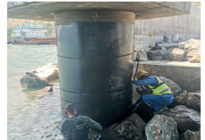
East Timor, Tibar Bay Port MarineProtect®-100 30 piers, DN 1800 (72")
