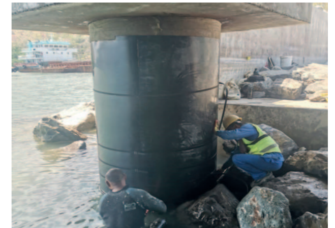
Osttimor, Tibar Container-Hafen MarineProtect®-100 30 Pfeiler, DN 1800 (72")
