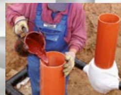
Sleeve pipe filling DENSO®-KS Mastic Hot Casting Compound
