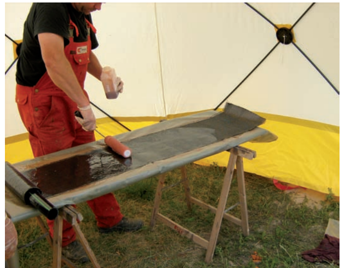
Fig. 3: Wet out of carbon mesh with 2-component Epoxy wet-out
