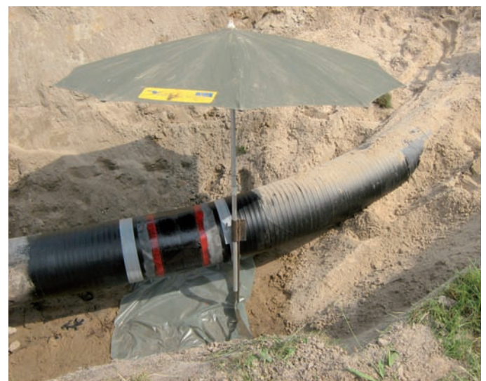
Fig. 5: Rehabilitated Pipe Section prior to application of corrosion prevention system
