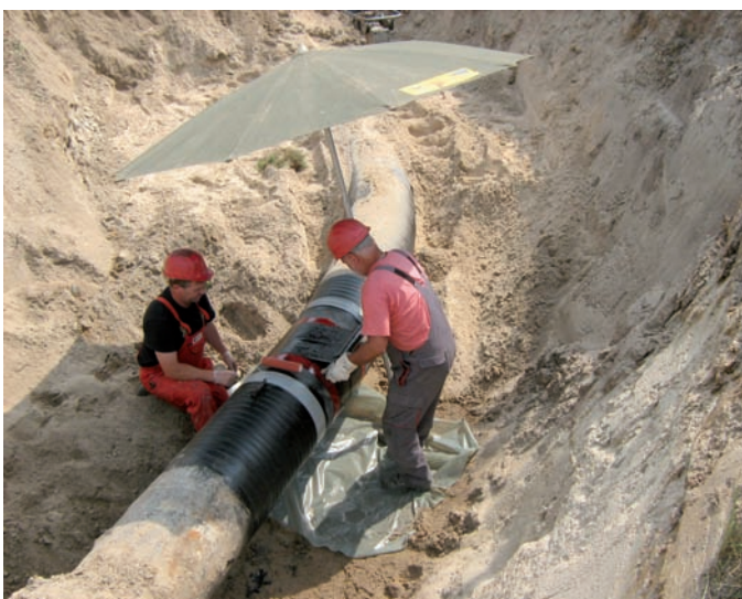
Fig. 4: Wrapping of saturated Carbon-mesh in several layers
