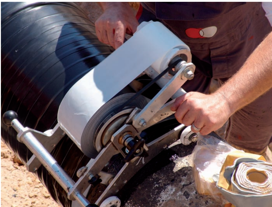
Fig. 6: Electrical isolation and corrosion prevention by applying 4 layers of DENSOLEN Tape
