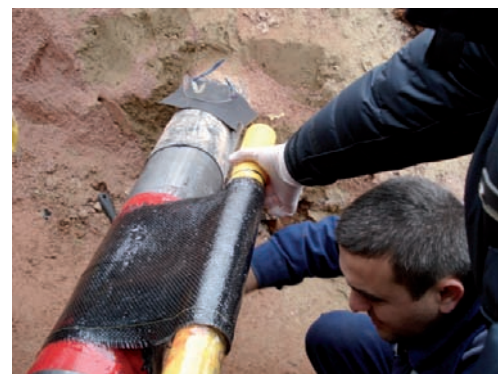
Fig. 1: Repair of a gas-pipeline section in Turkey with Black Diamond system
