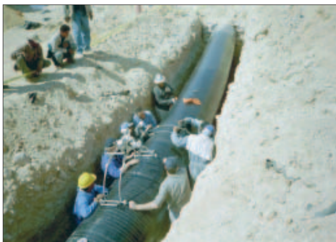
Fig. 2: Tape wrapping with DENSOMAT KGR Junior with extension arms
