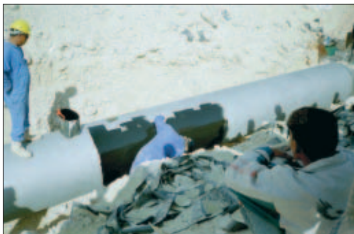
Fig. 1: Primer application by roller
