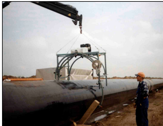
Fig 17 Easy mounting of DEKOMAT 11 wrapping machine on a 36" pipeline (girth weld insulation)
