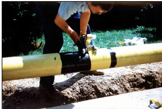
Fig 14 Tape wrapping with DEKOMAT 1 hand wrapping machine
