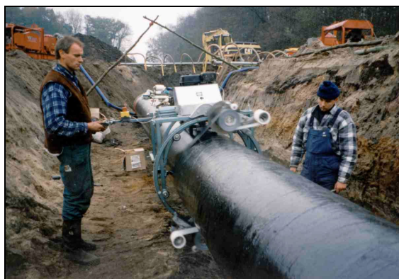
Fig 16 DEKOMAT 11 motor driven wrapping machine for coating refurbishment on a 24" pipeline
