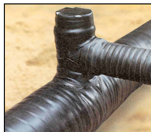
Fig. 9 Typical field of application for type 8b) two-tape system: Coating of weld-on branch line
