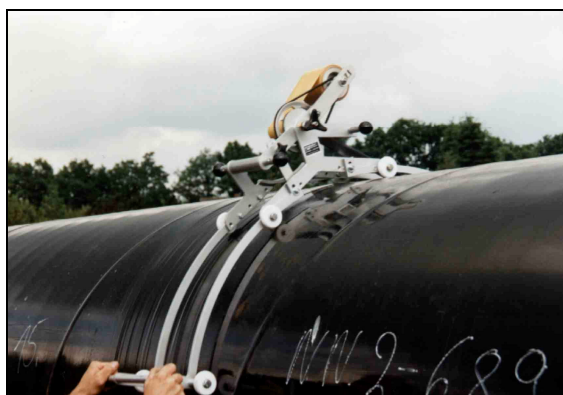
Fig 15 DEKOMAT KGR Junior hand wrapping machine with extension arms
