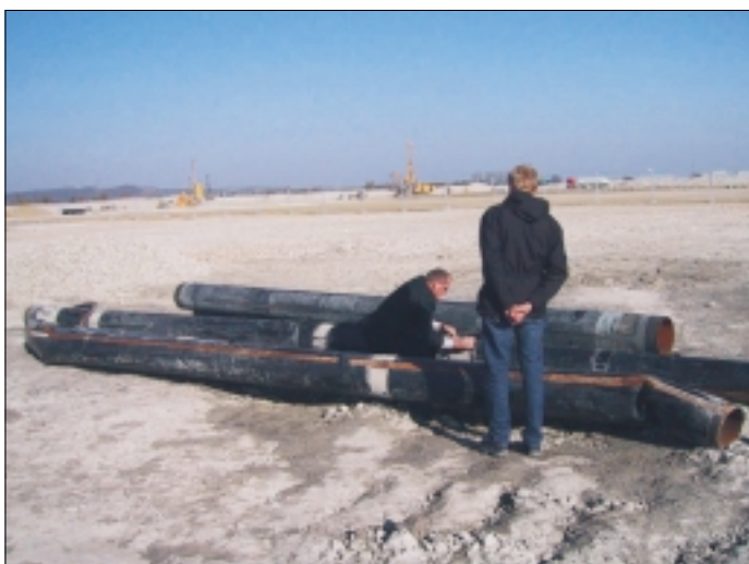
Fig. 2: Dismounted pipe segments DN 300
