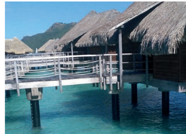
Polinesia Francesa MarineProtect®-2000 FD 1.019 pilotes, DN 300 (12")
