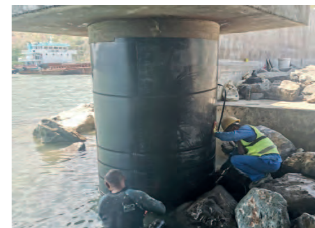
Timor oriental, port de conteneurs de Tibar MarineProtect®-100 30 piliers, DN 1800 (72")
