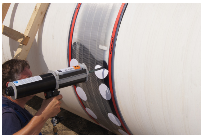
Figure 2. Application of DENSOLID-HDD with the two chambers cartridge.
