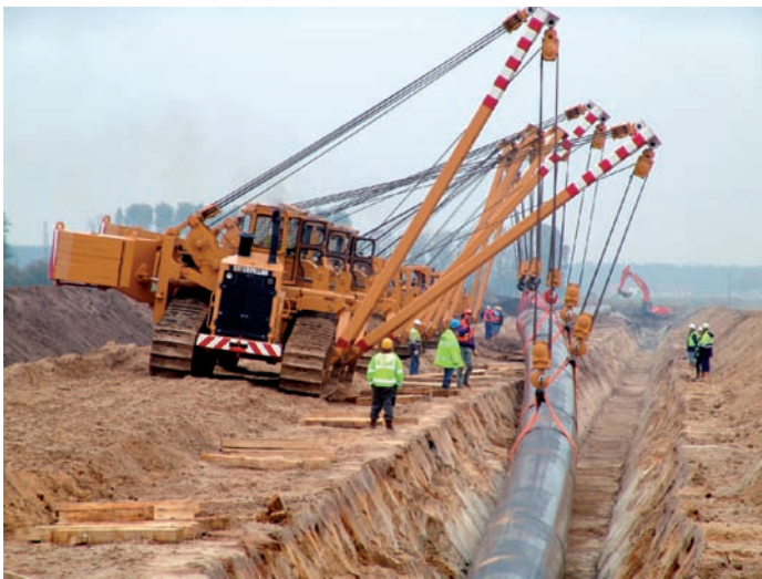
Fig. 15: Lowering of pipes into trench at OPAL
