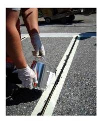
The surface temperature of the slit walls must be between +5 °C (+41 °F) and +40 °C (+104 °F). Always take care to observe the dew point. Any rising air bubbles must be removed (e.g. by painting over with a brush, or by
