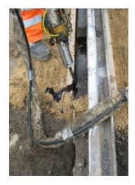
For rapid, high-quality preparation, a mechanical method is best, using a 2-component dosing machine.
