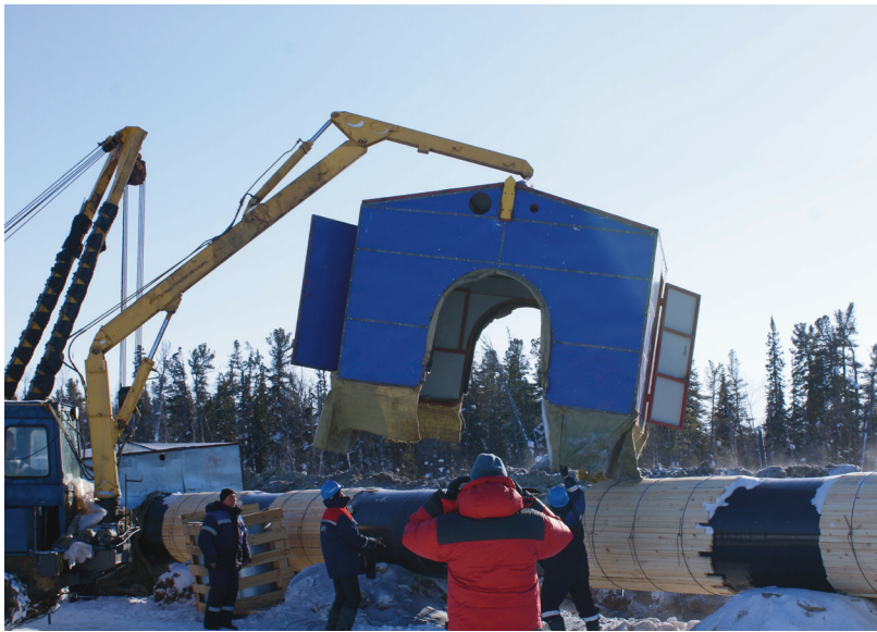
Figure 4. Welding tent at site.
